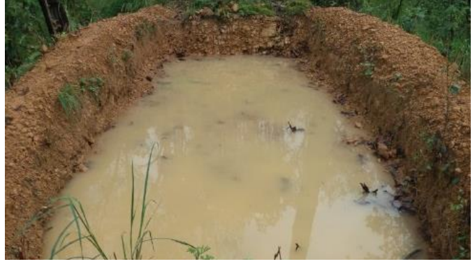
Recharge pond to collect rainwater
